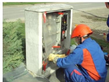
Fig. 2. Insulating glove method [2]
