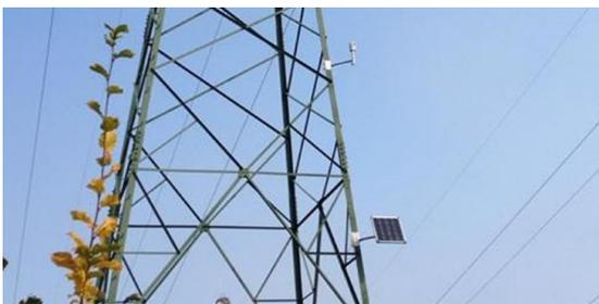
Fig. 7. Weather station installed on the high voltage tower [13]
