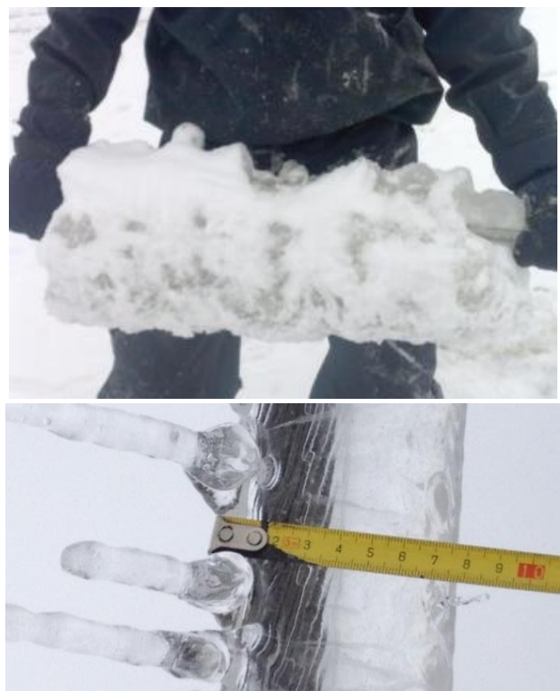
Fig. 1 Glaze ice on a conductor on the OHL 110 kV Cerčno – Idrija [1].
