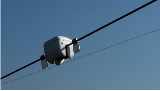
Fig. 5 Installation of OTLM SMART on the conductor.
