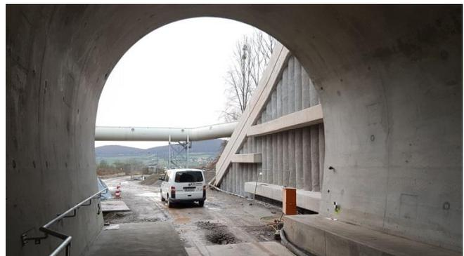
**Figure 1:** Tunnel portal with concrete surface and escape walkways.
