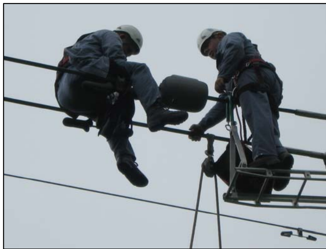
Fig. 1. Installation OTLM on conductors of OHL 400 kV
